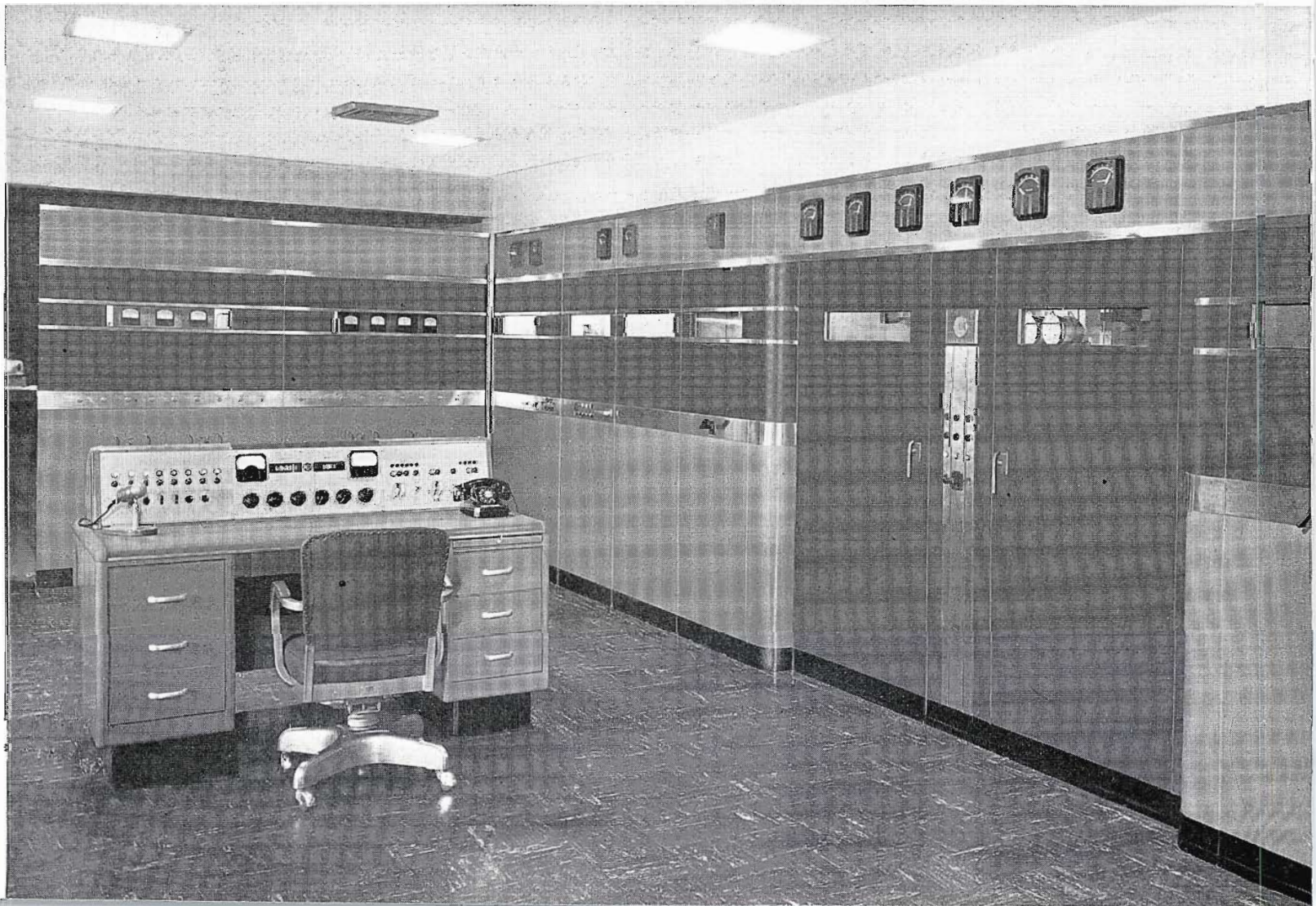
FIG. 1. 100-acre transmitting site of KRMG which is ideally located on a plateau not far from Tulsa. The land required no work prior to installation of the six-tower antenna system. Shown below is KRMG's new RCA 50 KW transmitter. Phasing equipment is built into the wall facing the supervisory console. Speech, monitoring and STL equipment is to the left of the console.
